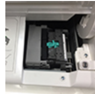
Ink waste tank maintenance
